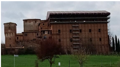
Figure 18.8: The fourteenth-century fortified granary of Cuna, south of Siena. The actual storage area is the tall part on the right. Other buildings behind and to the left housed laborers and soldiers who guarded the grain. Used until the early twentieth century, it then fell into disrepair and the roof is now being reinforced. Photo by the author.
