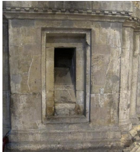
Figure 18.14: The opening of the grain chute in one of the piers of the ground floor. The grain would have been poured into the chute from the floor above and exited into a container held by a recipient. Photo by the author.
