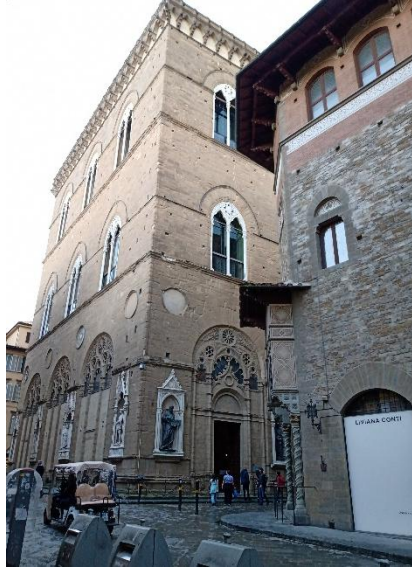
Figure 18.11: Orsanmichele has large windows on all sides opening onto the huge spaces of both upper floors. Photo by the author.
