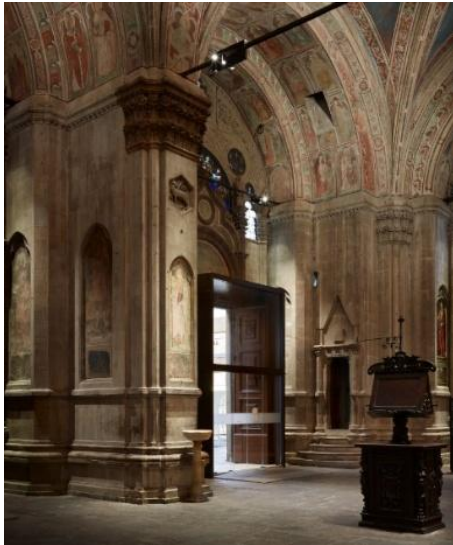
Figure 18.13: The door which leads to the staircase in the north/west pier or the ground floor of Orsanmichele. Note the opening above it, which could have been for protective purposes or for hauling up the grain. Photo by the author.
