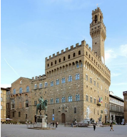
Figure 18.3: Palazzo Vecchio. The windows below the crenellations are in a covered walkway that is part of the defense system. The actual attic story of the palazzo is not visible. Francesco Bini, CC BY-SA 4.0 < https://creativecommons.org/licenses/by-sa/4.0/ >, via Wikimedia Commons.
