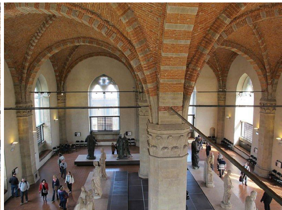
Figure 18.17: The luminous, vaulted upper floor of Orsanmichele. Note the opening to the grain chute in the lower part of the left pier. Photo by the author.
